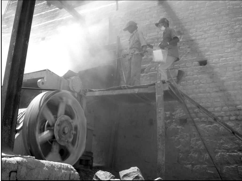
Picture 3: worker at the primary crusher chute
