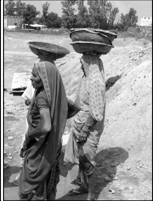
Picture 28: women transporting debris and gravel
