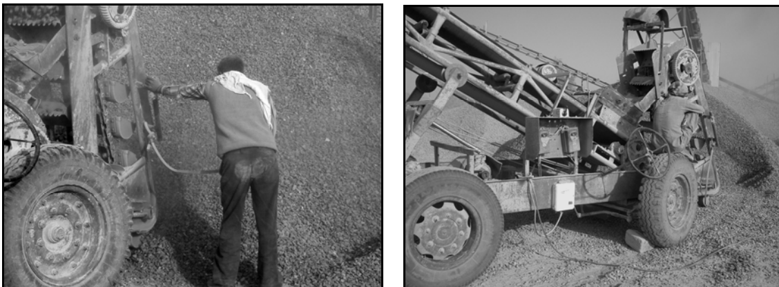
Picture 18: setting and adjusting the bucket conveyer for loading gravel
