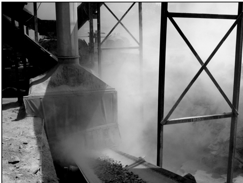
Picture 11: dust capture with dry ventilation and suction system
