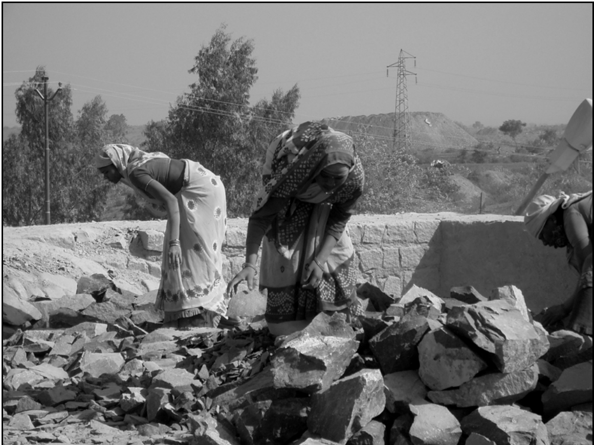
Picture 20: women leveling uneven surface on top of boulder pit by hand for truck traffic
