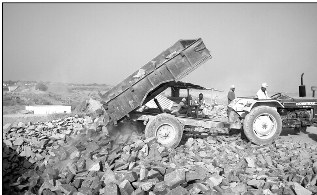
Picture 8: unloading boulders on top of boulder pit, workers resting (background)
