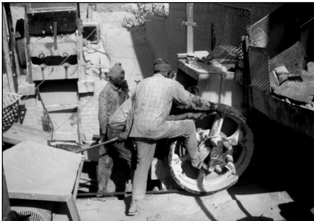
Picture 6: repairing the primary crusher, boulder chute on right
